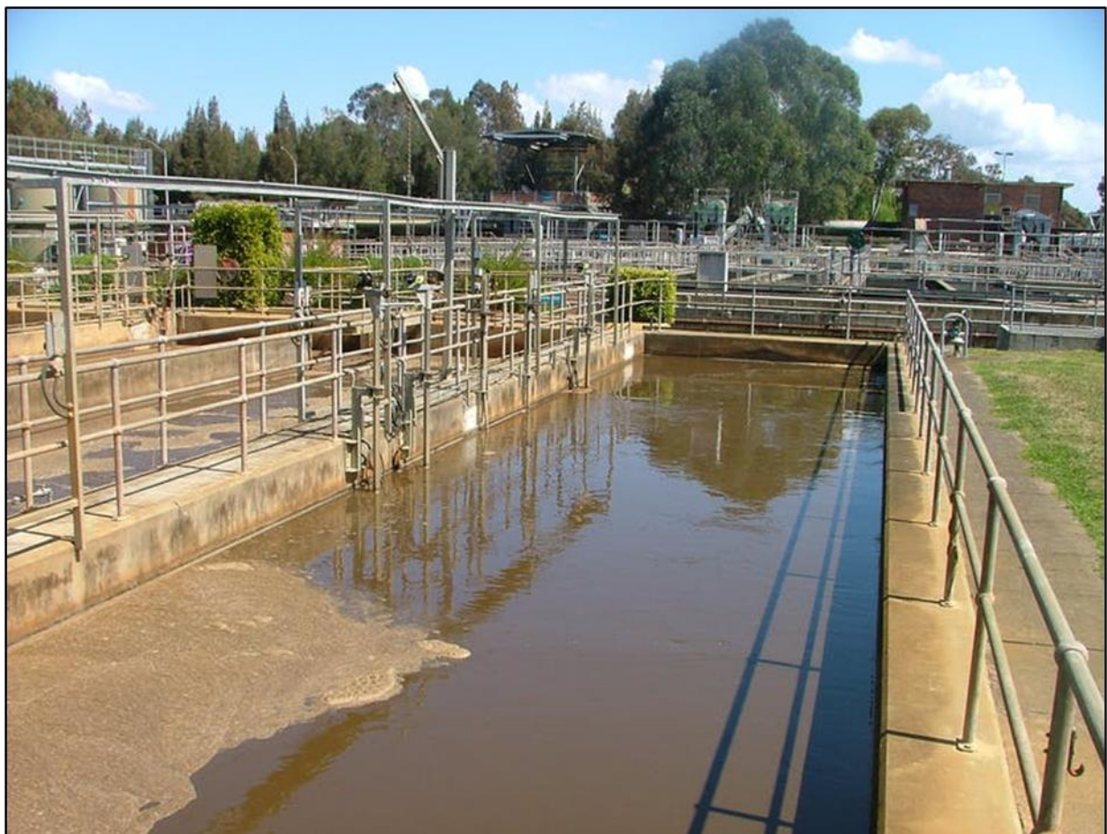
Figure 21. Sewage being treated at St Marys Sewage Treatment Plant. Photo Ian Wright.
